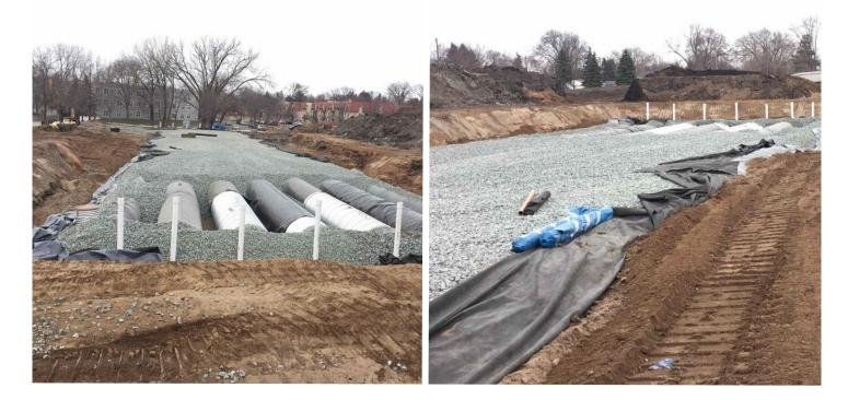
Images from top then left to right: Soil stabilization surrounding athletic field; 6-foot stormwater chambers; stormwater system covered (December 2020)
